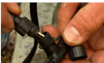
PLUG YOUR LIGHTS INTO THE CABLES
