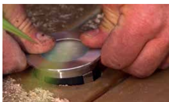
COMPLETE INSTALLATION OF LIGHTS
