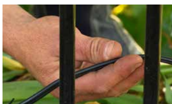
RUN LOW VOLTAGE CABLE
