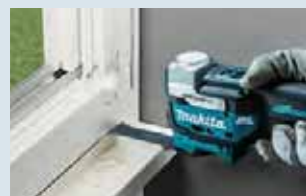
Removal of window frame
