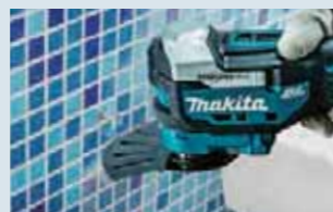
Routing joints on wall tiles
