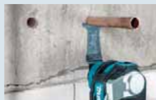
Copper pipe flush cutting
