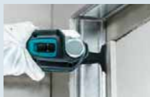
Door opening work
