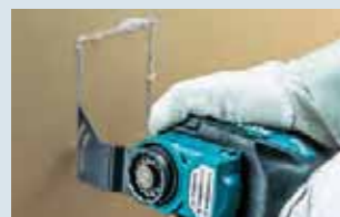
Cutting plasterboards
