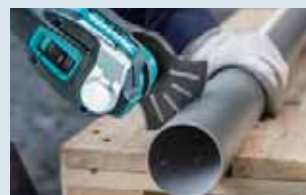
Cutting PVC, FRP pipes
